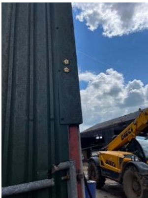
Unclear signage at Fulford Hall
